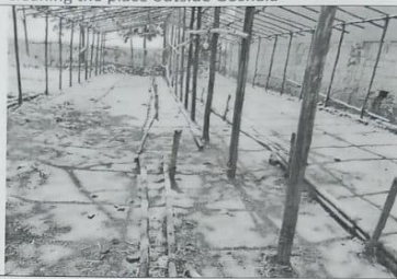
Cleaning the place outside Goshala (After)
